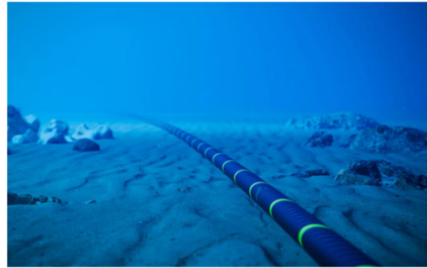
World's Longest Undersea Cable
